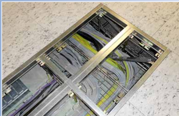
Frame area with exposed cable ducts
